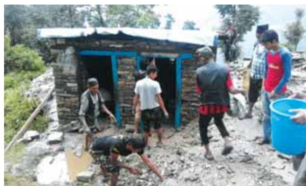
Demonstration of toilet construction during the mason training
