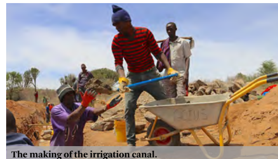
The making of the irrigation canal.
